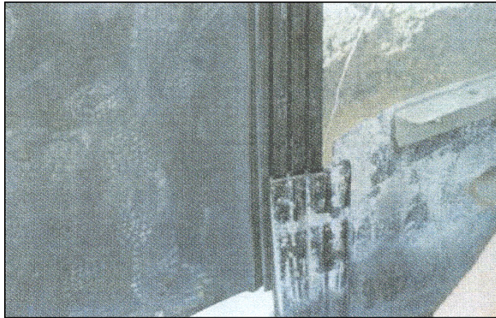
Figure 6 HDPE joint installation
