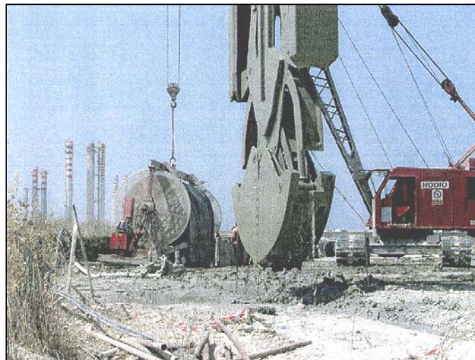
Figure 4 Excavation of the cut-off wall with clamshell (Granata and Crippa, 2006)
