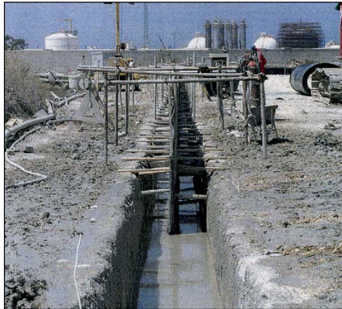
Figure 8 HDPE panels installed in the cut-off wall (Granata and Crippa, 2006)
