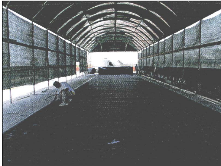
Figure 5 HDPE geomembrane cutting and joint welding (Granata and Crippa, 2006)
