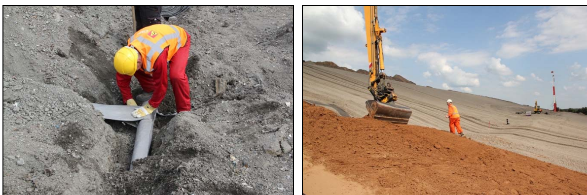
Picture 4: connecting the Multriwell Type H to the collector drain and covering it with a Trisoplast mineral liner
