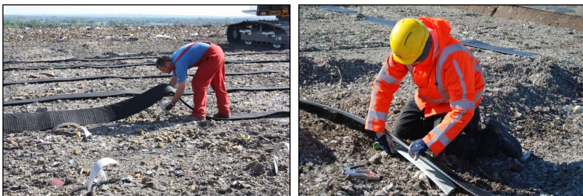
Picture 3: stapling the Multriwell type V to the type H
