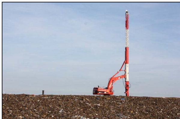
Picture 1: Excavator with Sticher.
